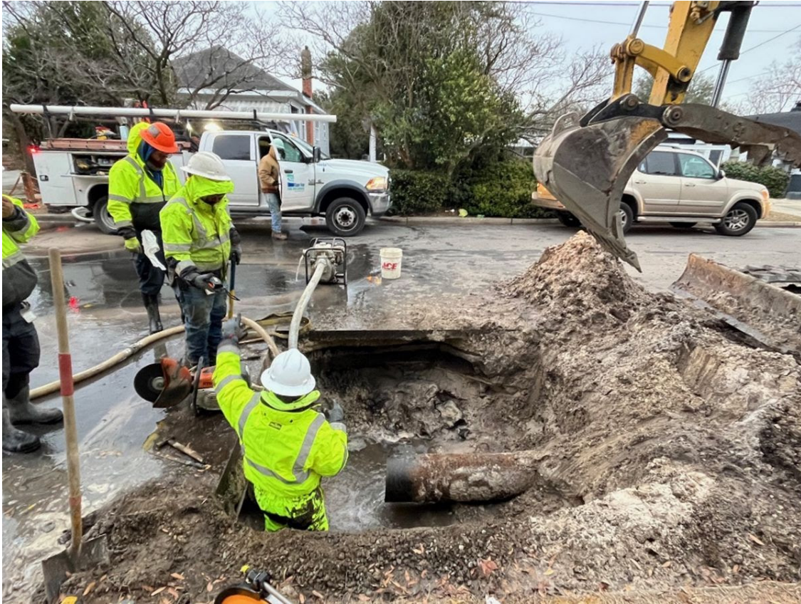
CFPUA Distribution and Construction staff repair a broken water main on South 11th Street, January 21, 2025.
