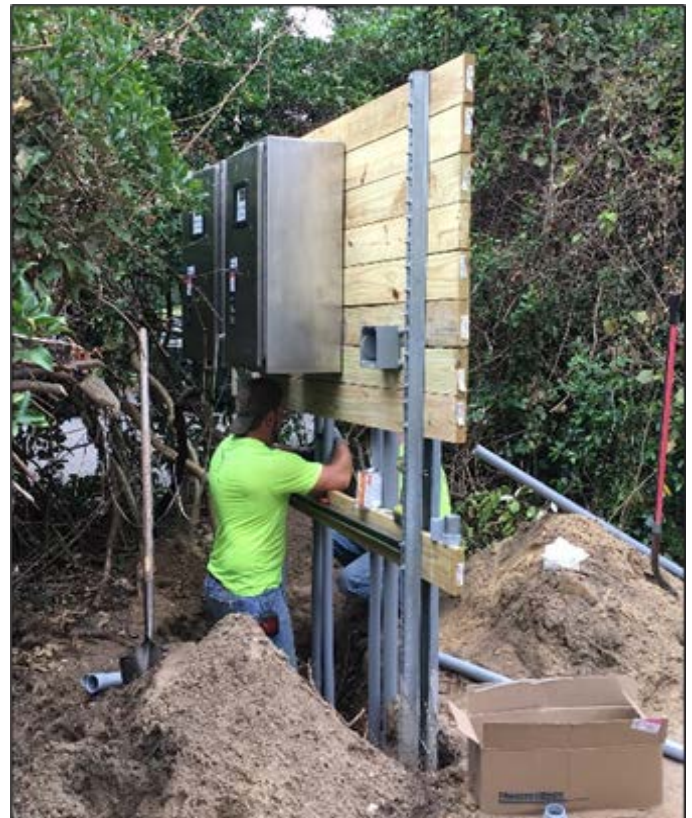
Raising Electrical Control Panels
