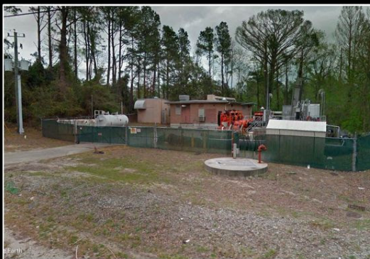
Pump Station #34 BEFORE
