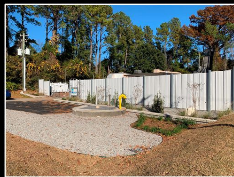
Pump Station #34 AFTER
