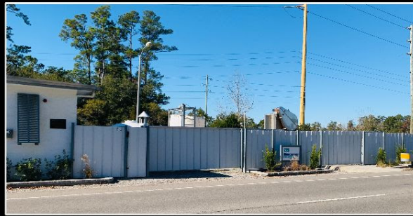
Pump Station #35 AFTER
