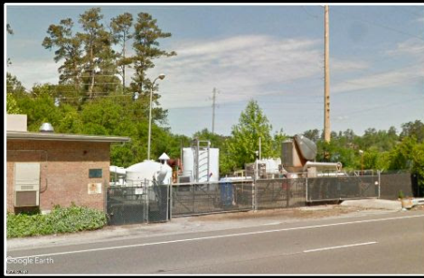
Pump Station #35 BEFORE
