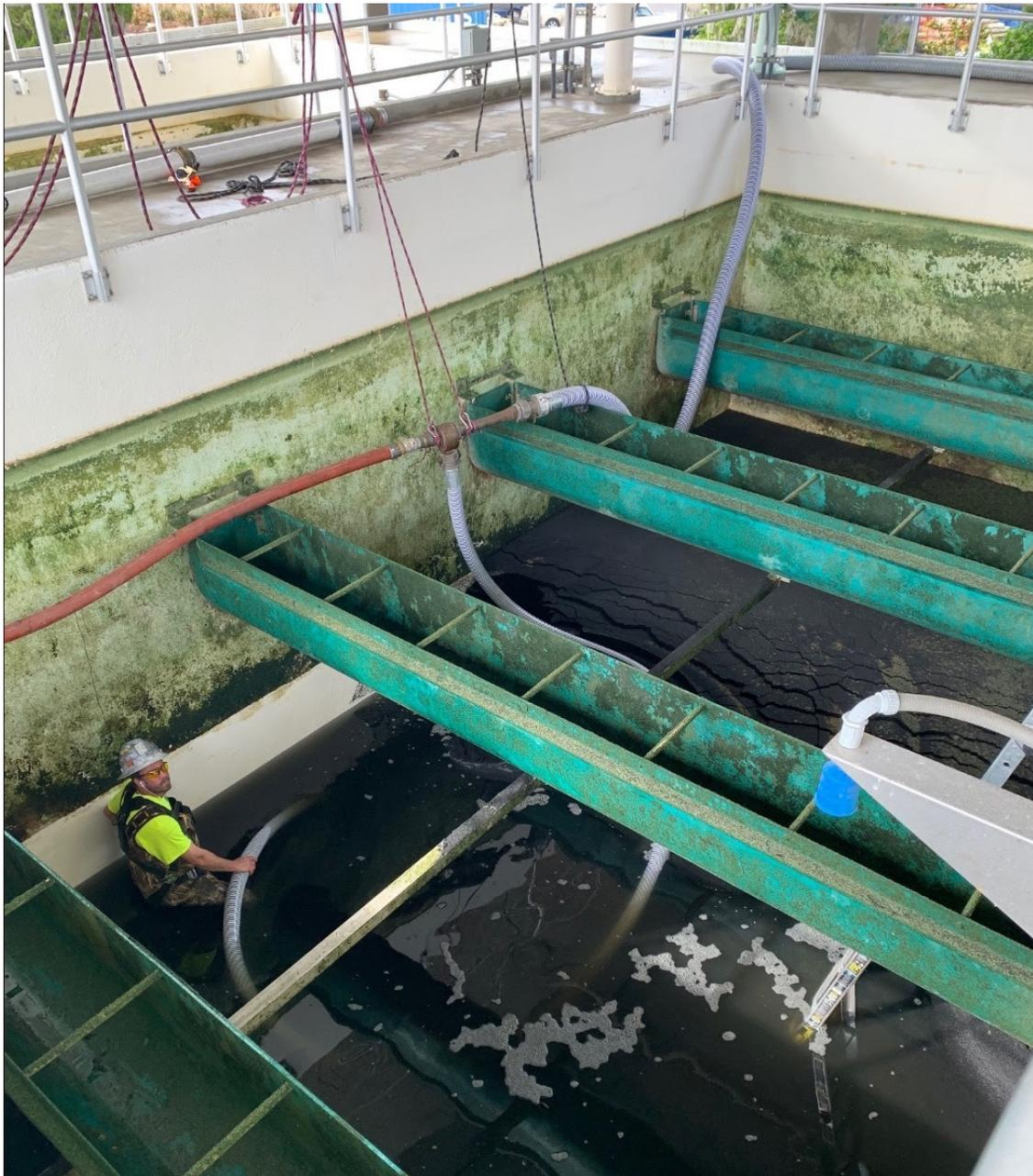
Filters at CFPUA's Sweeney Water Treatment Plant will get an additional change-out of Granular Activated Carbon (GAC) as construction continues on new deep-bed filters at the plant.
