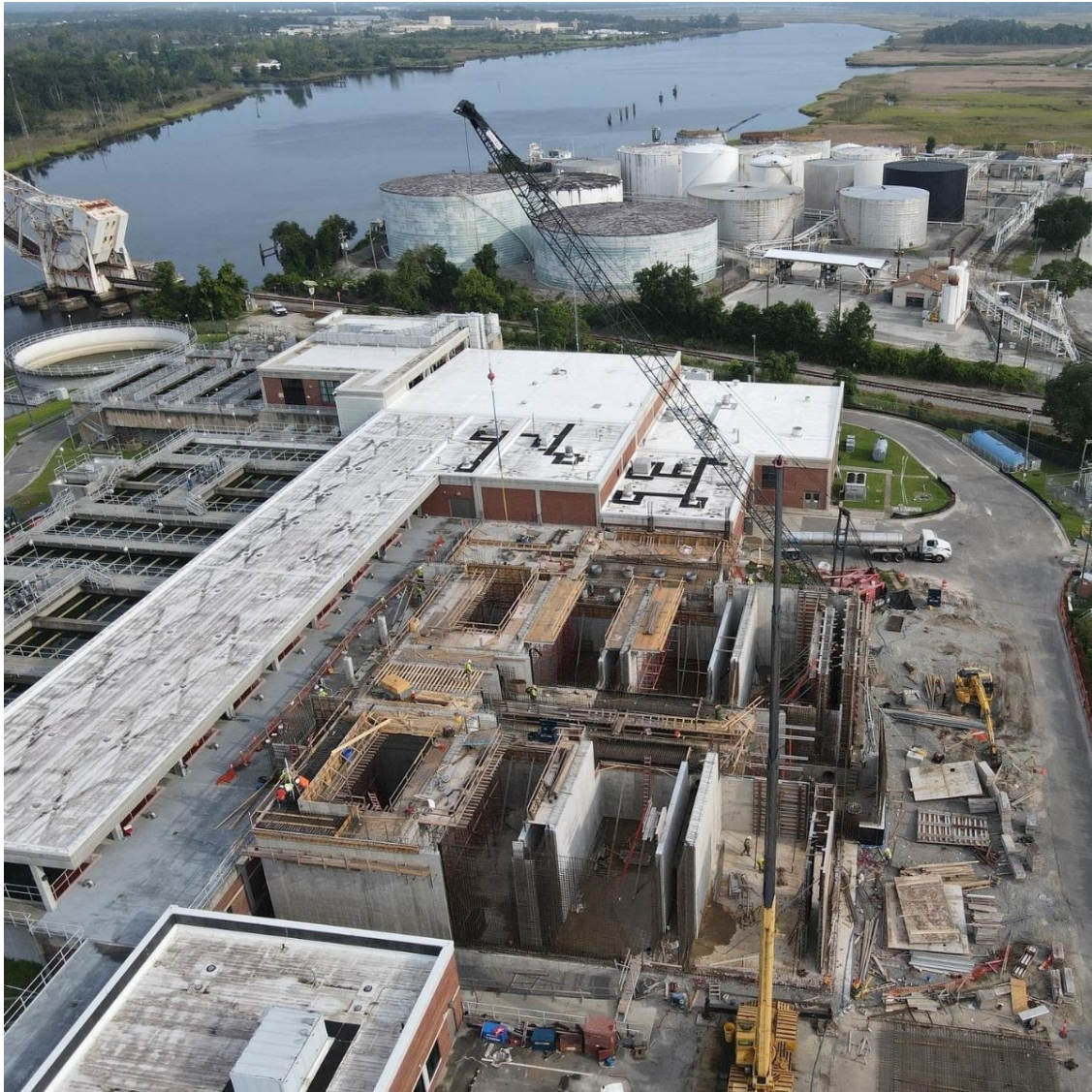
Construction on the new filter facility in August 2021
