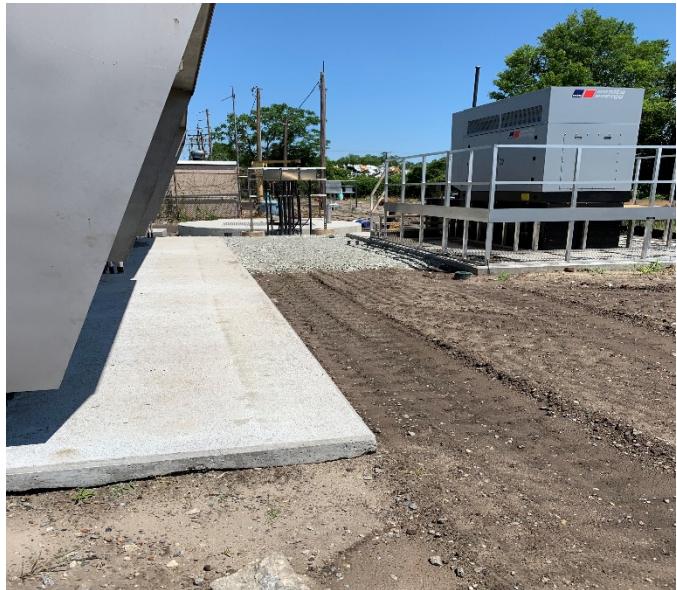
Figure 1: PUMP STATION 13 DAWSON STREET
