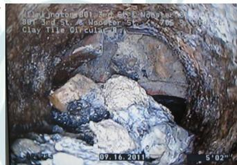
The crawler recorded this portion of clay sewer pipe that had collapsed.
