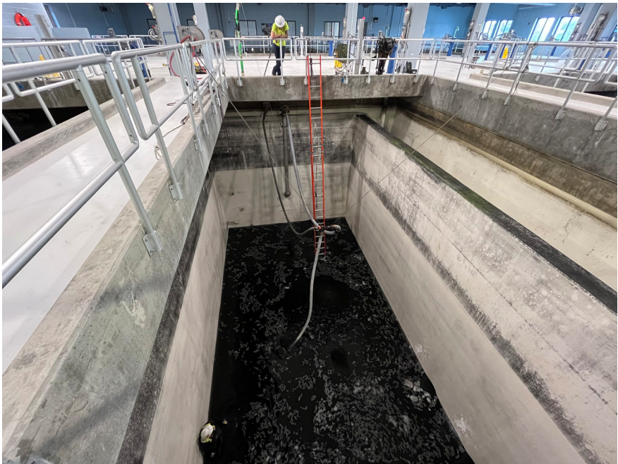
Crews removing GAC media from a filter at CFPUA’s Sweeney Water Treatment Plant in 2023.
