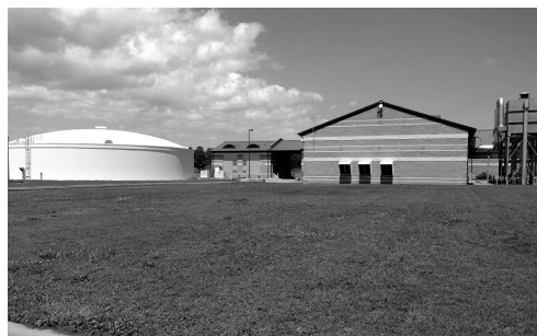
Michael E. Richardson Water Treatment Plant
