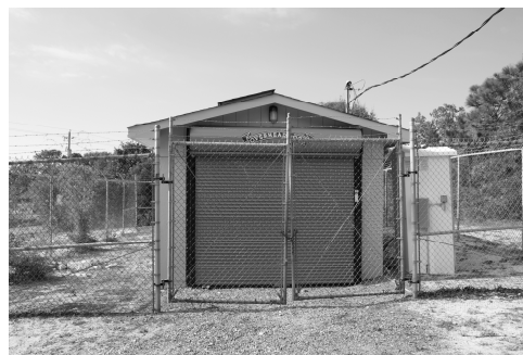
Well #MH1 - Cathay Road
