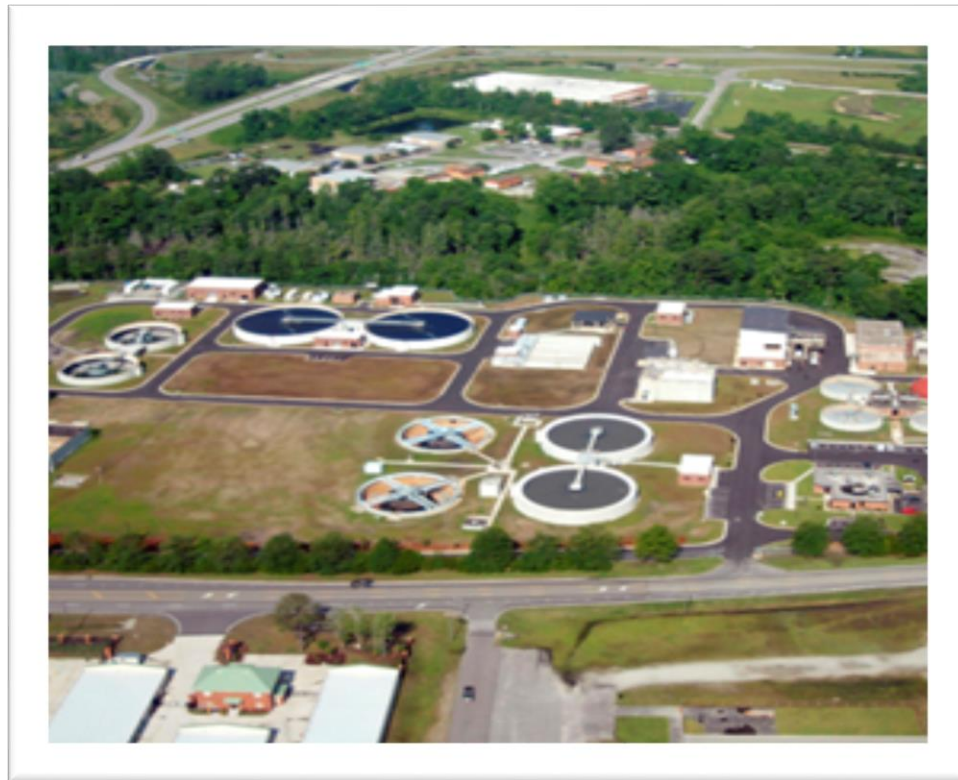
Northside Wastewater Treatment Plant
