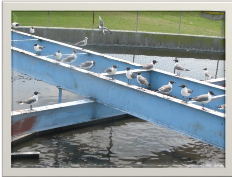
Photograph by Jacqueline Valade, Southside Wastewater Treatment Plant
