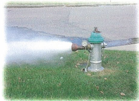
Flushing of Hydrants to ensure water quality within the system
