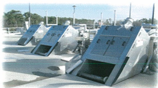
Northside WWTAP Aeration Basin
