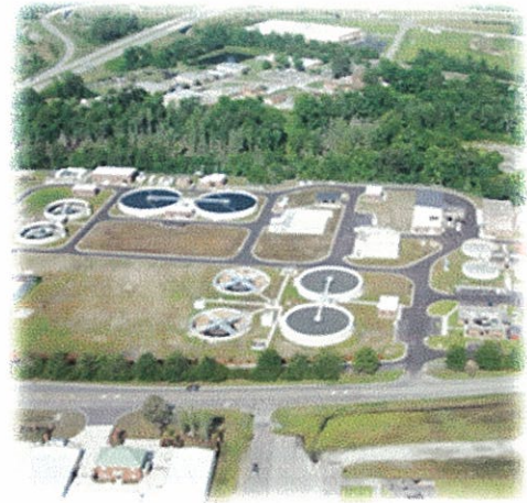
Northside WWTP Aerial
