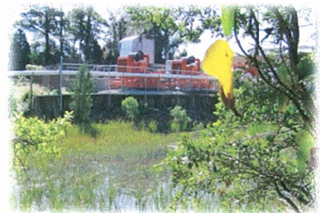
Bradley Creek Pump Station
