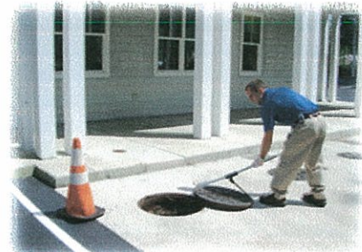
Compliance Staff inspecting grease trap
