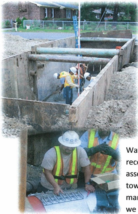
TOP: Construction Staff working on lines in Trench Box
