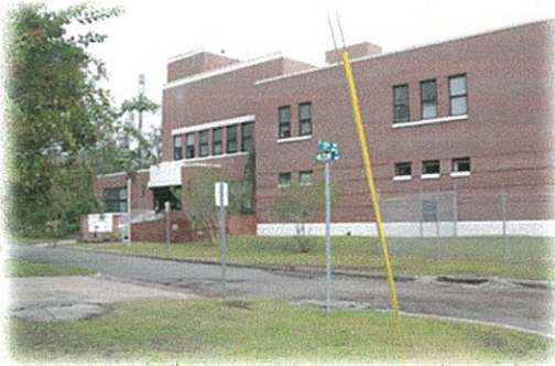
Sweeney Water Treatment Plant and Authority Laboratory
