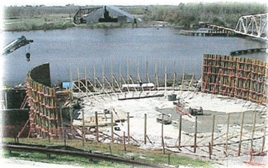
Sweeney Upgrade Project
