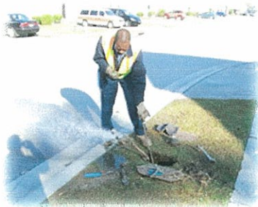
Meter Services employee repairing meter
