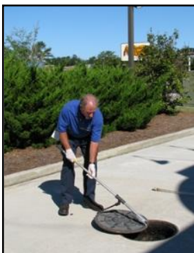
Compliance Officer inspecting an interceptor
