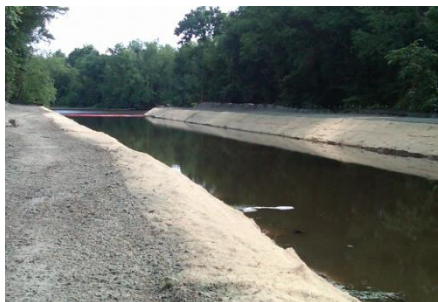
Channel dredging and bank restoration at King's Bluff Pump Station
