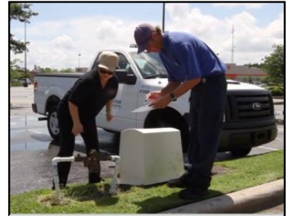
Compliance Officer Reviewing Backflow Prevention Records
