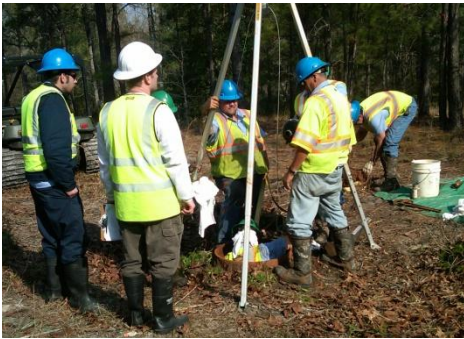
EMS Auditors observing Right of Way / Heavy Equipment personnel replace an air relief valve along the raw water line
