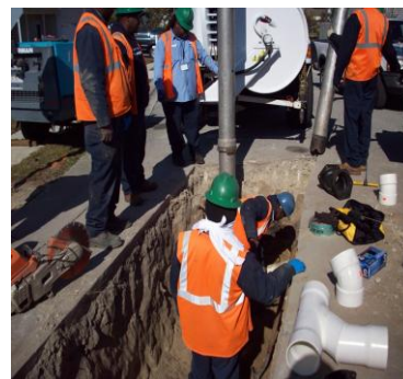
Crew installing a new service
