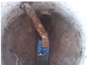
Manhole Before Rehabilitation
