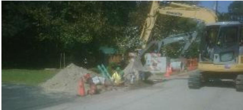
Hydrant Replacement Project
