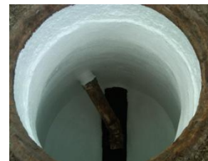
Manhole After Rehabilitation
